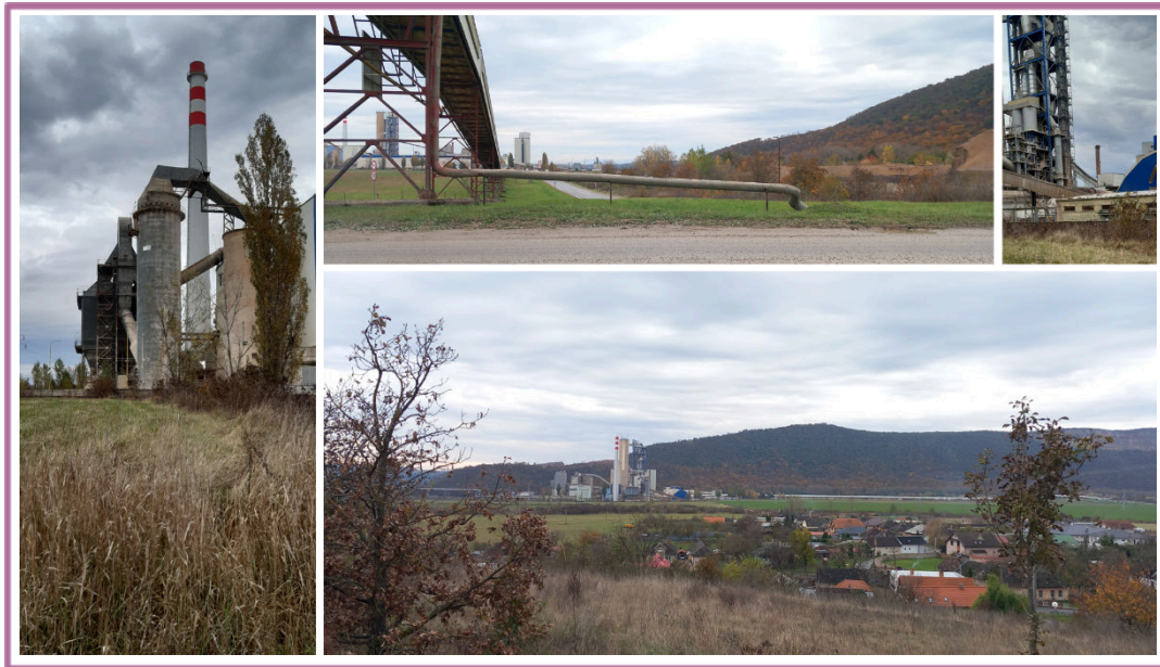
Figure 1 - The cement kiln Turňa nad Bodvou
