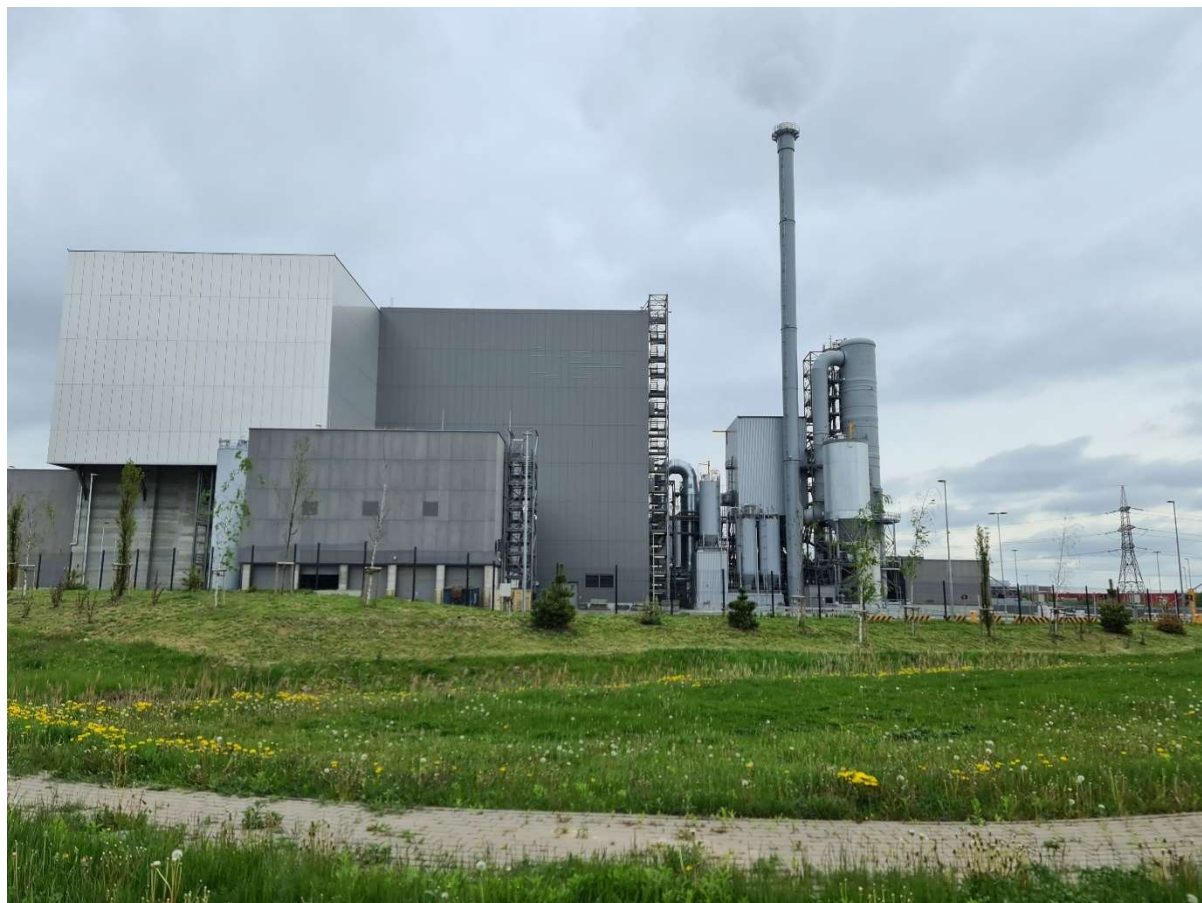
Figure: UAB Kauno Cogeneration Power Plant, (WtE)
